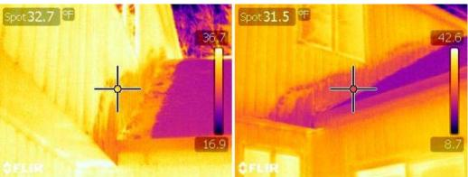
Moisture is soaking into the rear siding. Recommend diverting rain water from the upper
